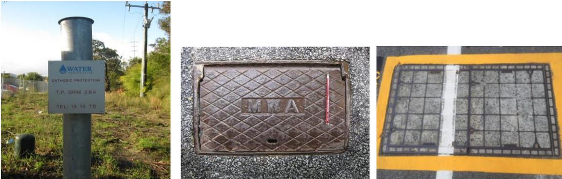
**Cathodic protection test point (left); valve cover (centre); trafficable sewer maintenance cover**
