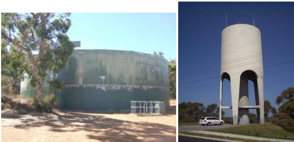
**Examples of a Ground-level Water Storage Tank and a Water Tower**
