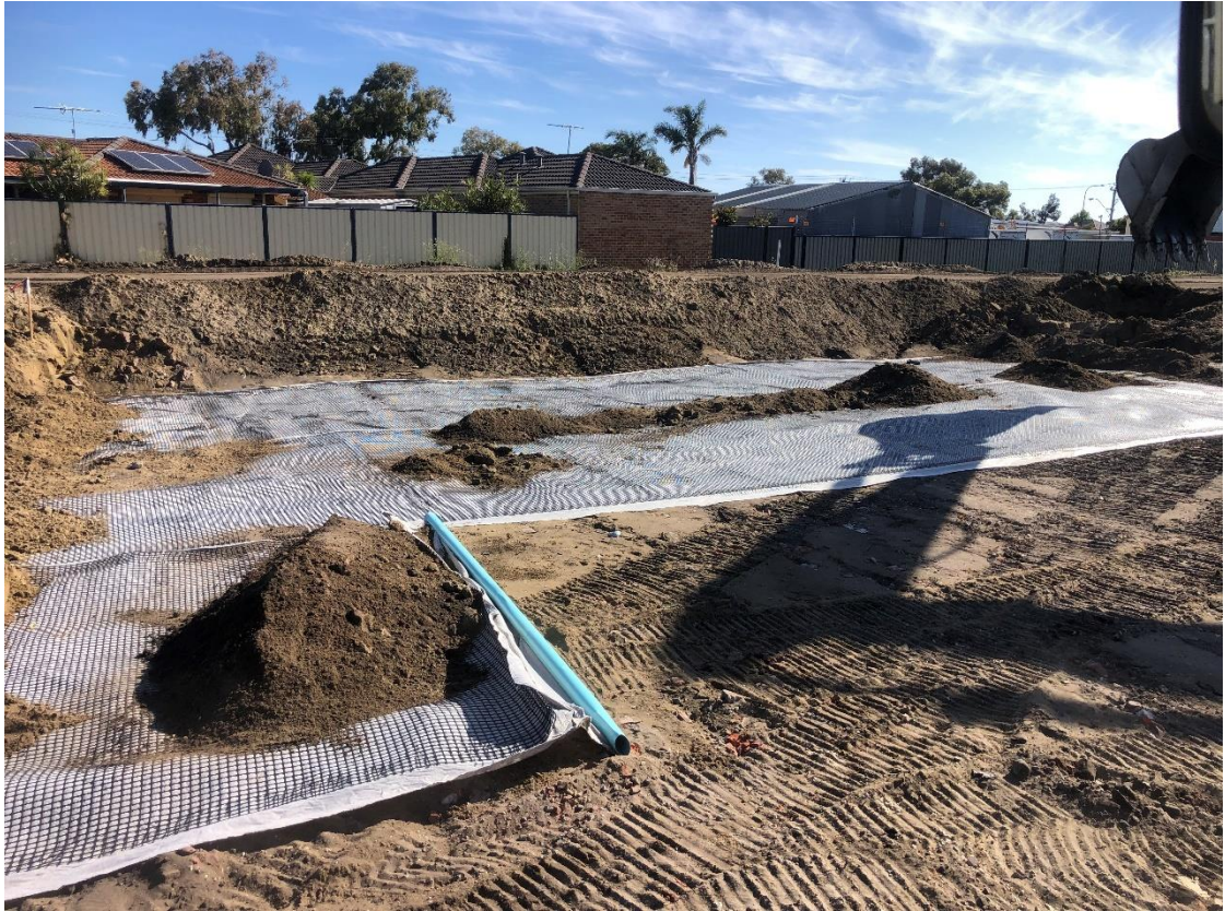
Photograph 1: Geotextile laid above the containment cell.
