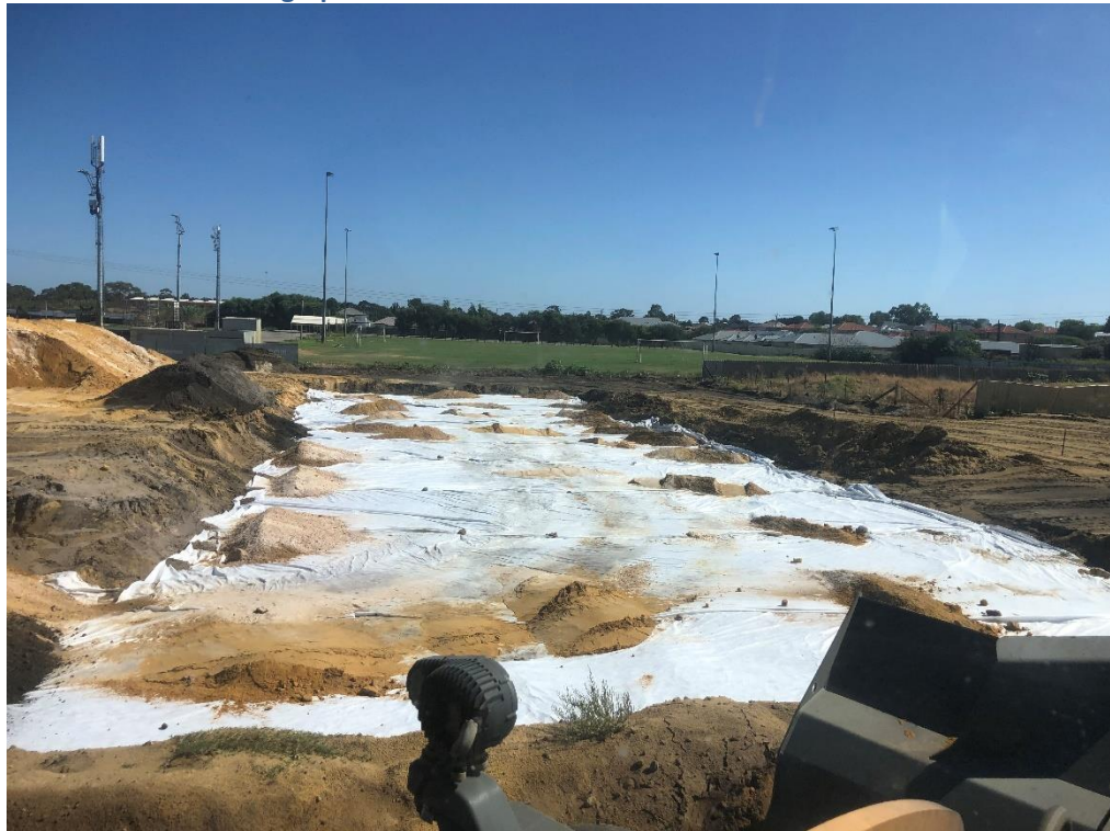
Photograph 2: Geotextile laid above the containment cell.
